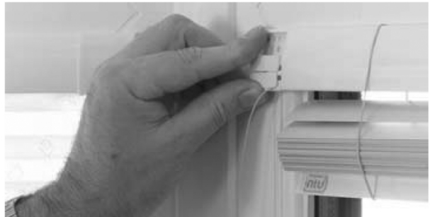
7. Stick blind onto frame leaving rubber band around blind.
