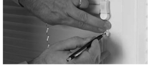
B2. Remove pulley cover, lightly tension lift cords down window side, mark position to fix pulley.
