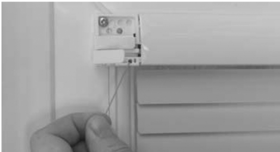
12. Remove rubber band. Carefully release locking gate. Pull cord to tension approx. equal on both sides
