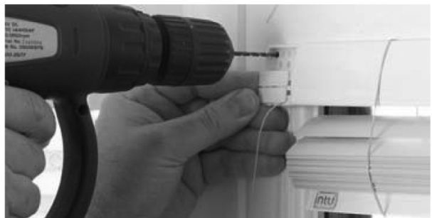
8. Drill Ø2.5mm holes 2 off on each side.
