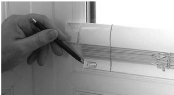
4. Using blind, mark positions for the cord grommet holes.
