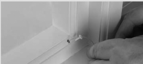
A4. Push cord knot into brass insert, push grommet into brass insert, aligning groove to cord.
