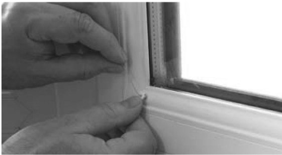
11. Holding button, pull cord tight to secure
