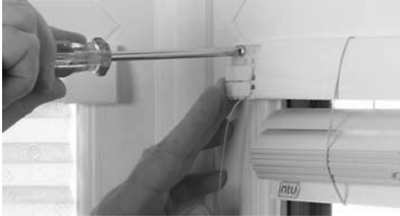
9. Hand screw fixings.
