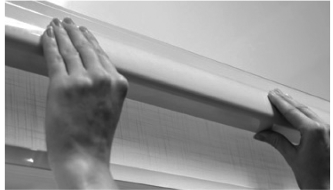
15. The blind can now be pushed fully home onto brackets.
