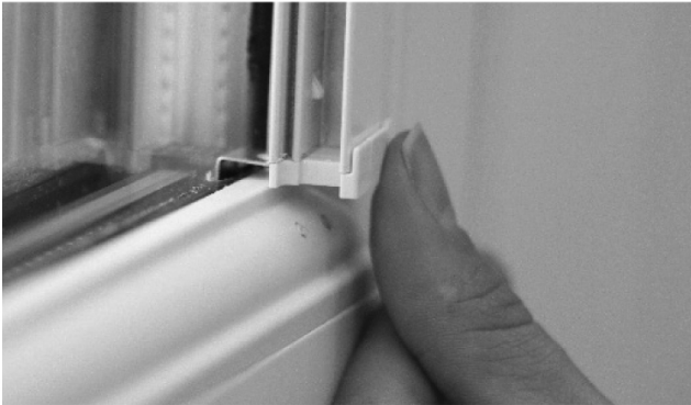
13. Engage the side extrusion bottom bracket into the bottom corner fixing bracket.
