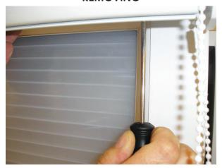
To remove the blind, push the lip of the bracket at the back of the cassette upwards using the head of a screwdriver. This will free the back of the cassette. Carefully remove to avoid damage to the blind.
