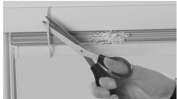
16. Snip off the rubber bands and carefully lower the slats to the bottom frame.
