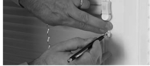
B2. Remove pulley cover, lightly tension lift cords down window side, mark position to fix pulley.
