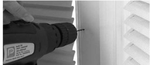
B3. Drill Ø2.5mm hole 1 off.
