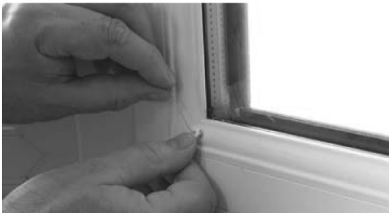
11. Holding button, pull cord tight to secure
