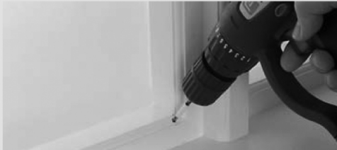
A2. Mark position as outlined in step 4 (over leaf). Drill Ø4mm hole to depth of 10mm.
