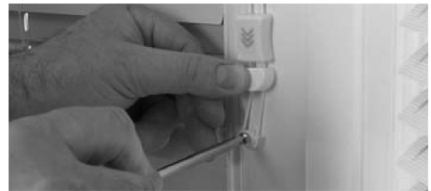
B4. Hand screw fixing
