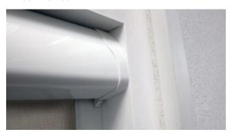
10. Headrail fascia should be pushed fully on ensuring locks are engaged on both sides.
