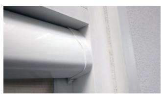
8. Side profile can then be clipped home onto the top corner fixing bracket.
