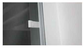
Position relevant number of side profile clips according to the drop of the blind.
