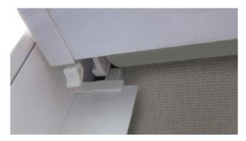
5. Insert one side of fabric and corresponding bottom bar endcap into side profile and push headrail onto top corner brackets on both sides. N.B. Do not push blind fully home onto brackets.
