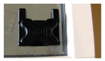
2. Insert bottom corner fixing bracket behind rubber bead, repeat on opposite side.
