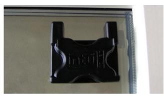
1. Using fitting tool, insert top corner fixing bracket behind rubber bead, repeat on opposite side. N.B. Bracket positions must be manually adjusted when fitting side extrusions and headrail fascia based on frame shape and size.
