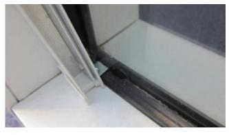
3. Locate the profile bottom endcap over the bottom bracket, once fitted use side profile to position bottom fixing bracket.
