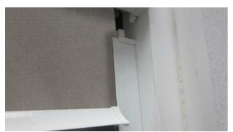
6. On opposite side, tilt bottom bar to open position and slide profile over bottom bar endcap and fabric ensuring both are located within the fabric channel on the side profile.
