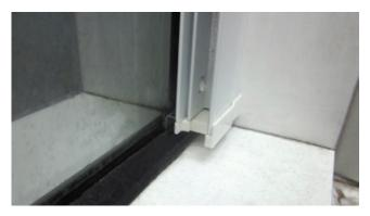
7. When the side profile is pushed all the way up and is in position, engage the side profile bottom bracket into the bottom corner fixing bracket.
