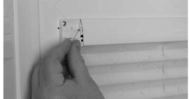
13. Press locking gate closed to secure cord. Cut-off excess cord leaving 100mm min. Tuck through hole in endcap.
