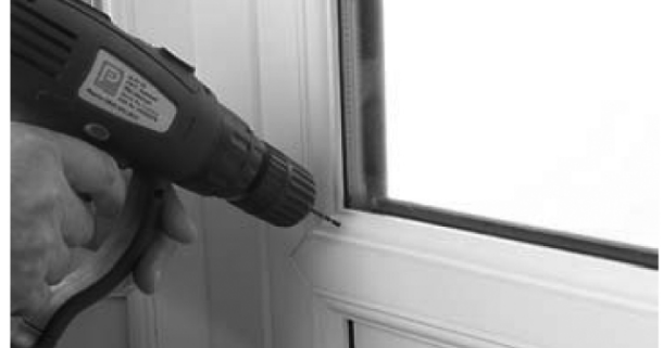
5. With the drill at 90° to the surface, drill Ø2.5mm hole 1 off on each side.
