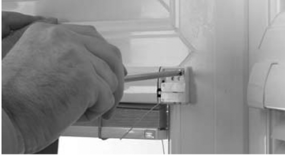
9. Hand screw fixings.
