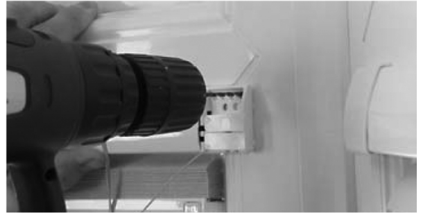
8. Drill Ø2.5mm holes 2 off on each side
